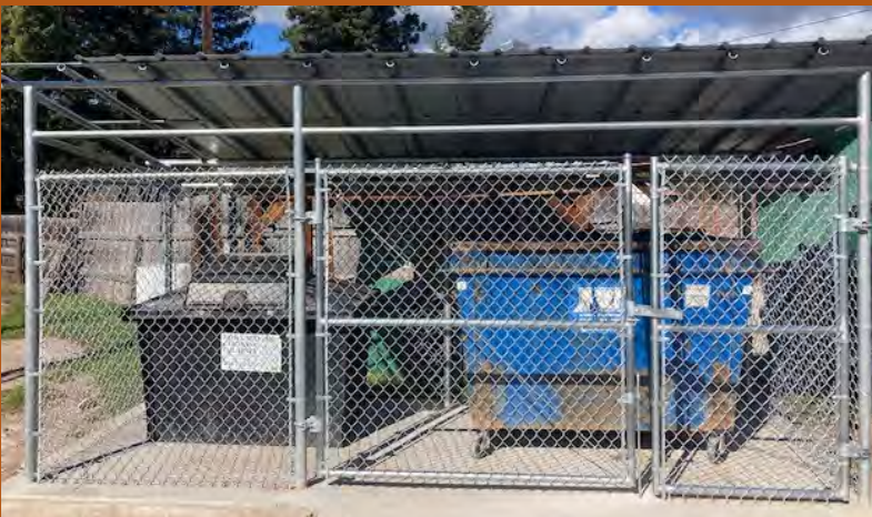
Top: Bear-proof electric fencing enclosure located behind the Ice Cream Place; Bottom: Bear-proof fencing with metal roof cover located behind the Filling Station.
